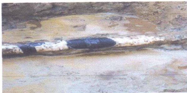
REPAIR WORK DONE BY NAOC REPAIR TEAM
